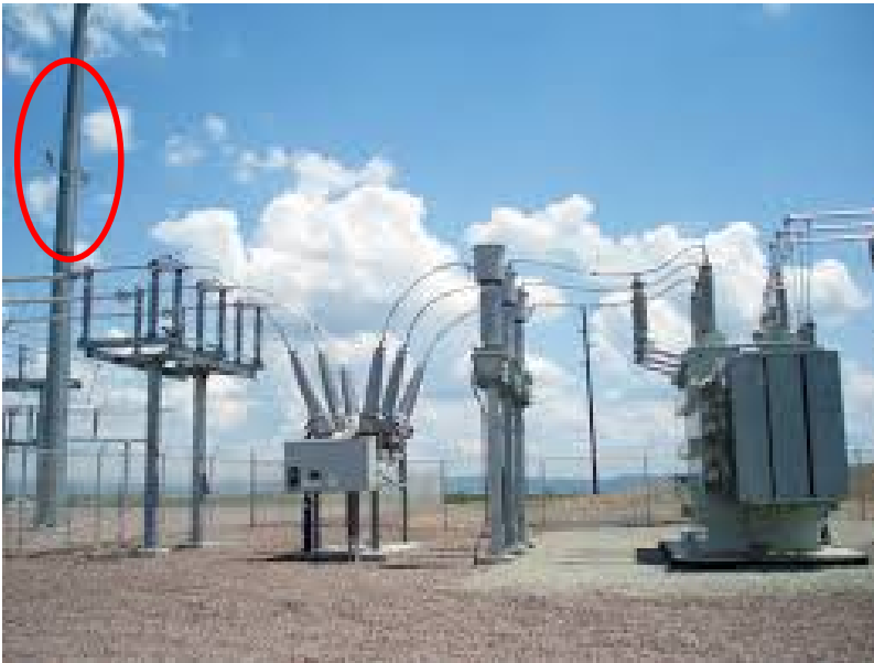
Figure.5 – Typical Pole Mounted Lighting for Substation Lighting
