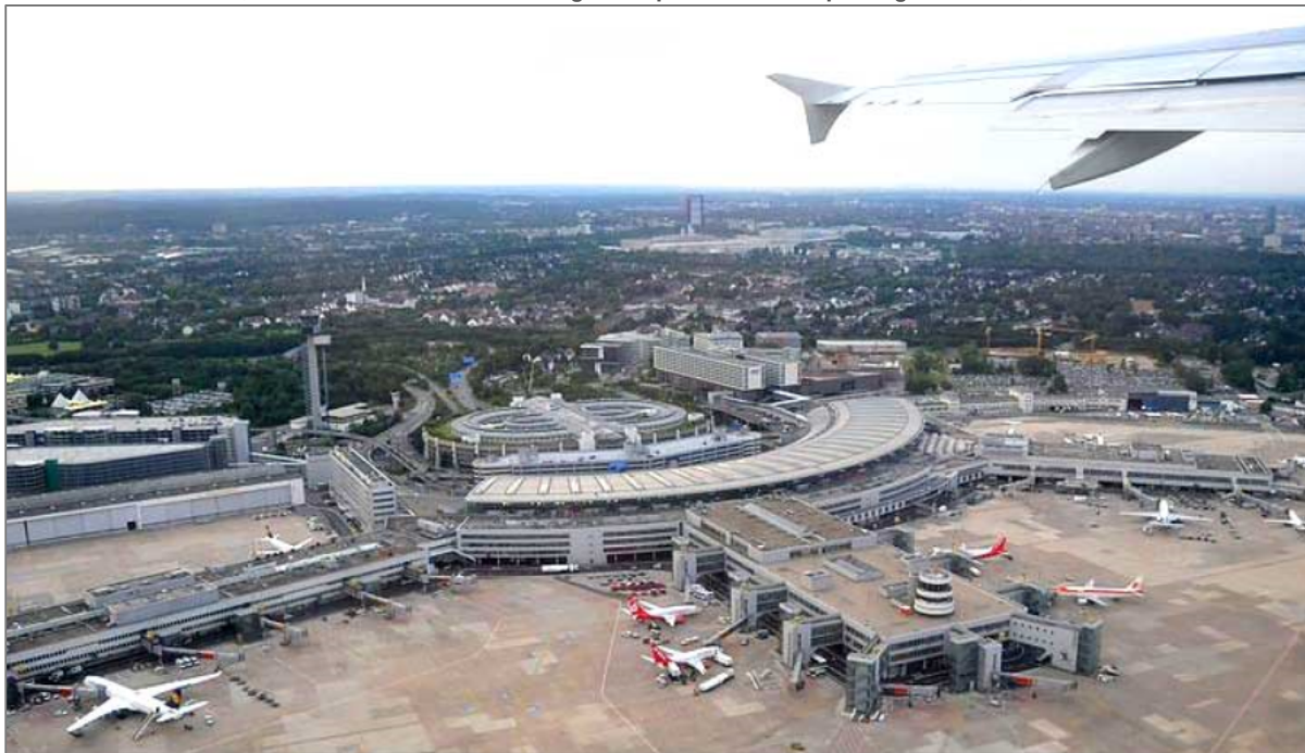
Figure 31 – 8,400 solar panel array on roof of Dusseldorf International Airport, 2011 Source: Solar Choice, www.solarchoice.net.au/blog/solar-panels-near-airports-glare-issue , 2013
