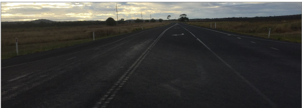
Figure 19 – Gore Highway at intersection of Yarranlea Road, looking Eastwards Source: Site Visit, June 2016
