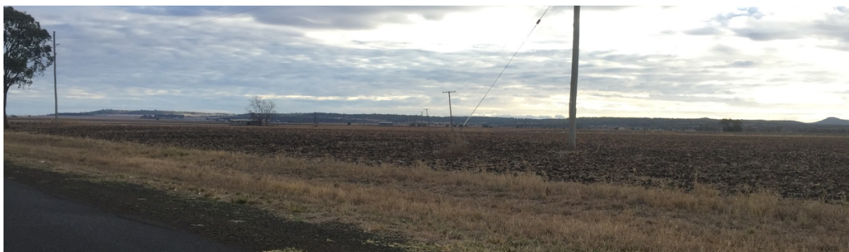
Figure 3 – View of proposed Solar Farm from SW corner of subject lot on Yarranlea Road looking NE Source: Site Visit, June 2016
