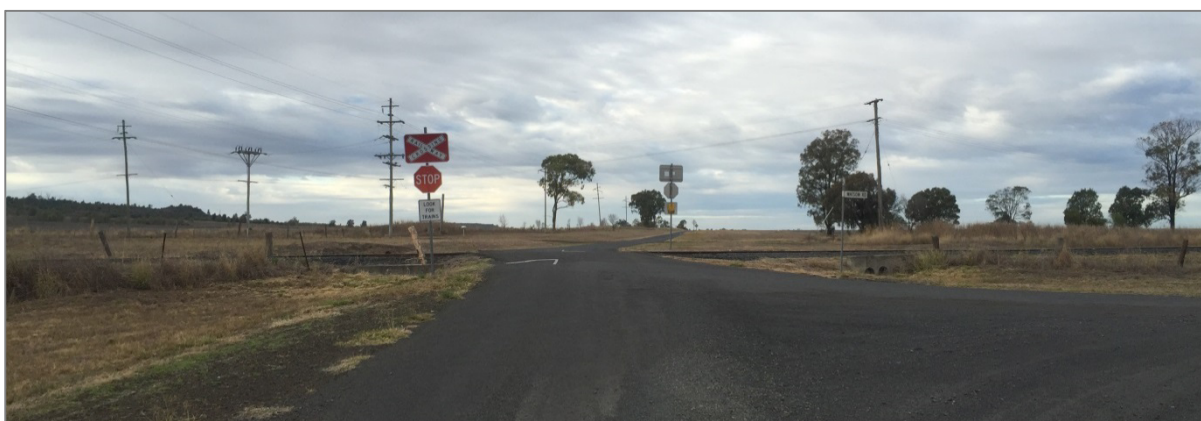
Figure 25 – Intersection of Yarranlea Road with Railway line, heading southwards away from subject lots Source: Site Visit, June 2016
