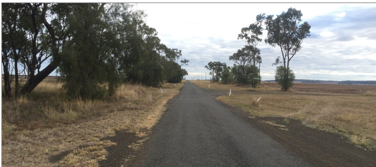
Figure 6 –Yarranlea Road and Murlaggen Road intersection looking Northwards Source: Site Visit, June 2016
